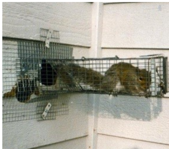
Figure 1. Squirrels can damage homes and other structures. This squirrel has been captured in a live trap near the damaged site.
